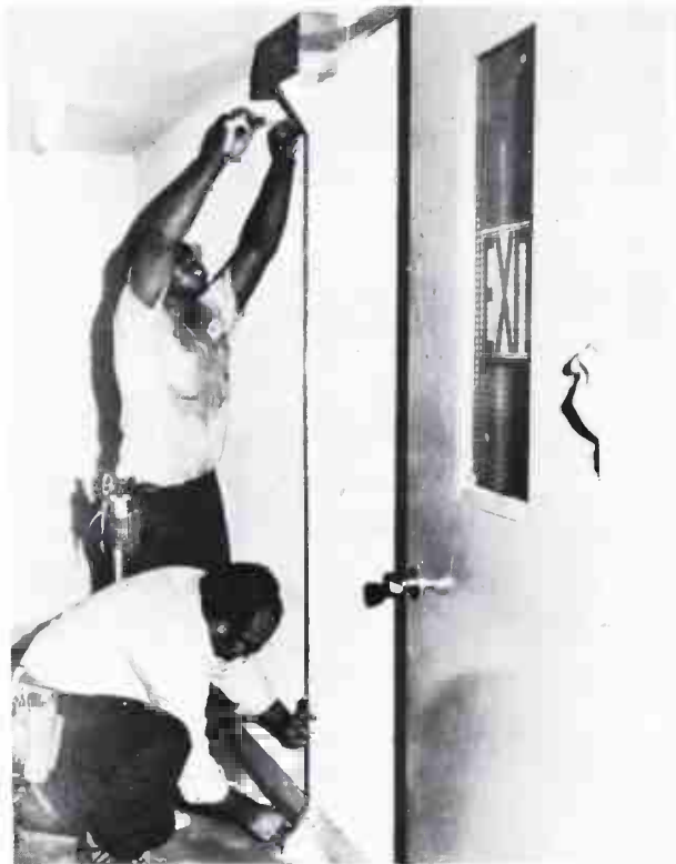
Vertical risers are installed between floors in fire stairwells. Aluminum ducts conceal the cable.
