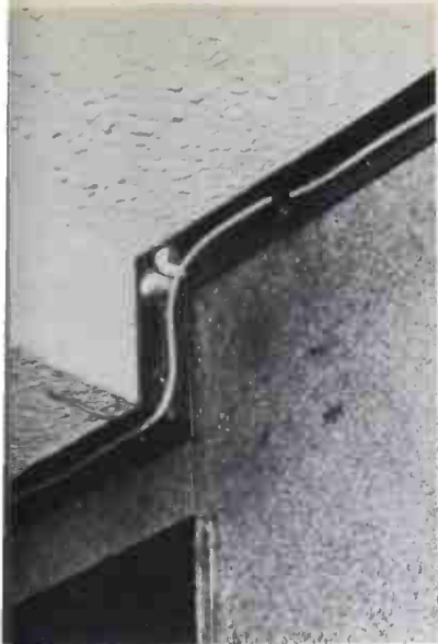
Molding channel is installed inside public hallways. A molding strip snaps into place concealing cable.
