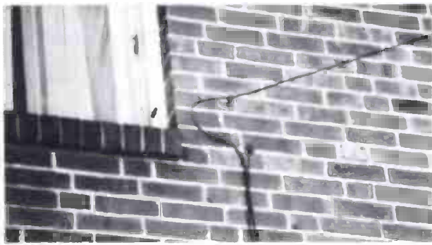
A fatigue loop is also put in drop cable at house attachment.
