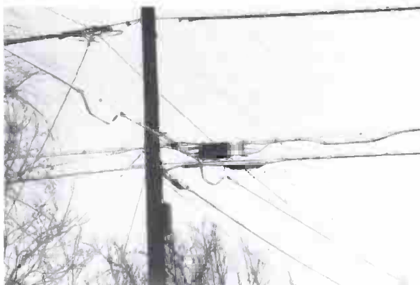
Note how expansion loops are formed. Other construction details are shown.
